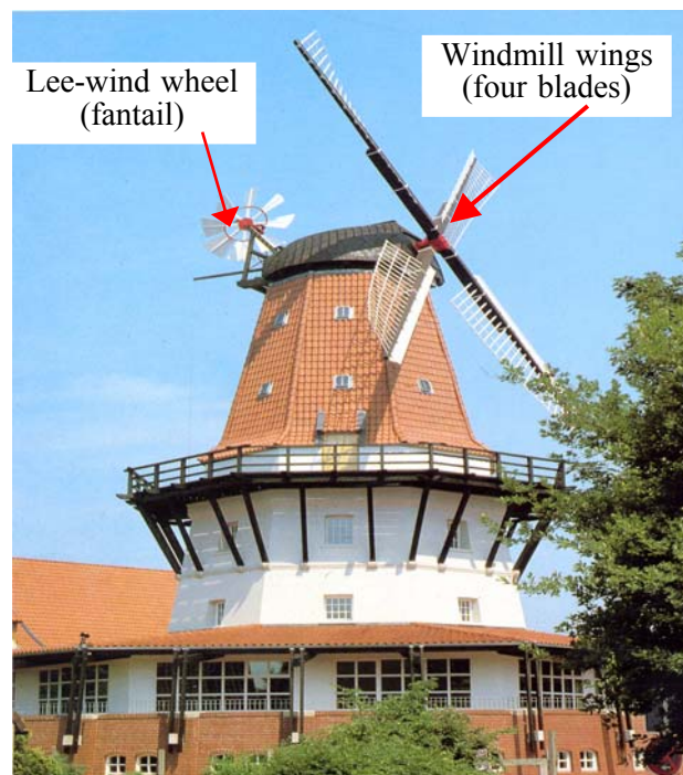
Figure 3.27: Historical windmill with a lee- wheel on the tower cap in the town Peine, Germany.
