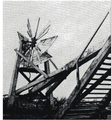
Figure 3.26: An eight-bladed ground-level fantail attached to the tailpole.
