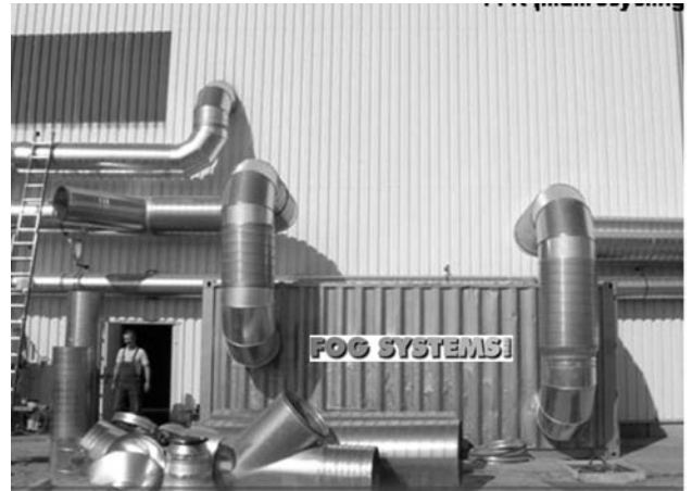
Figure 7: Setup with standard container (20 Feet), air flow 30 000 m 3 /h, water 300 l/h and 40 Nozzle; picture: Fog Systems
