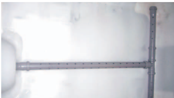
Abb. 12: Rohrdrainage - Drainage pipe.
