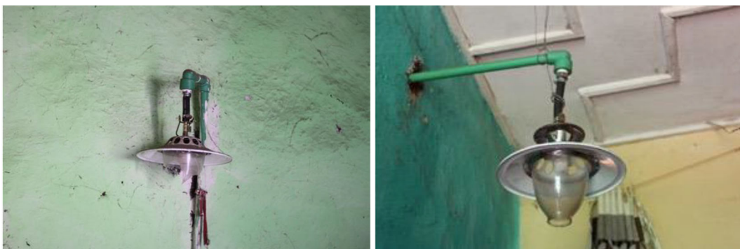
Picture 6 A broken biogas lamp compared with a functioning biogas lamp. Source: Own
