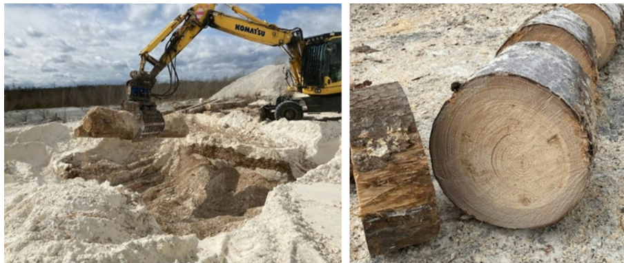
Fig. 8 Removal of in-ground stored Norway spruce logs
